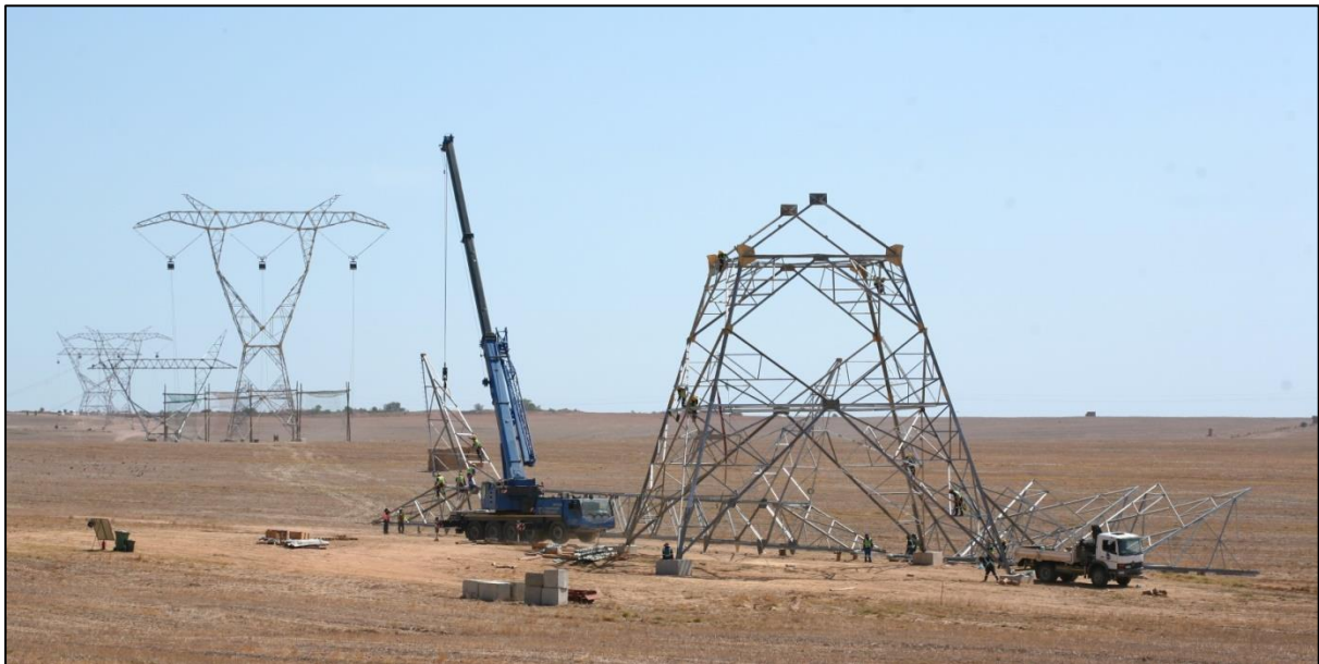
Construction of pylons along the Kappa-Omega 765kV line, illustrating the disturbance footprint typical of pylon construction. Although this is local and largely superficial, it can extend well beyond the actual footprint of the pylon tower.
