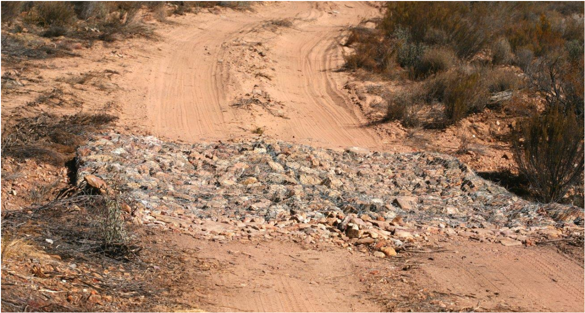
Rocky bed gabions used to facilitate river and drainage line crossings on the Kappa-Omega 765kV line. Similar gabions should be used on the Juno-Gromis line for river crossings.
